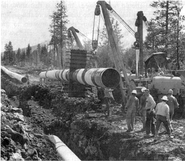
FIGURE 3.10 Gate Valve Being Installed on the TransAlaska Pipeline
